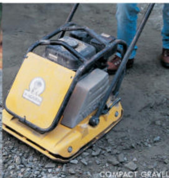
AFTER EXCAVATION, APPLY GRAVEL LAYER
